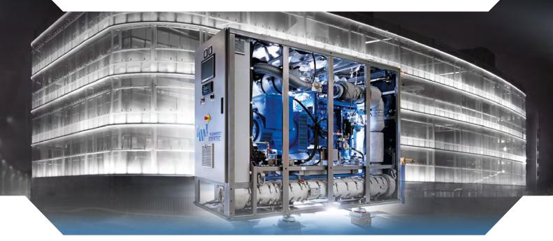
ENERGIN® CHP units produce heat and electrical power at the same time. The heat recovery is from engine jacket water, exhaust, lube oil and the first stage of mixture cooling.
